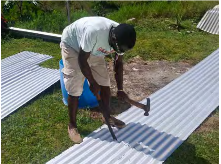
Cutting roof panels with a machete
