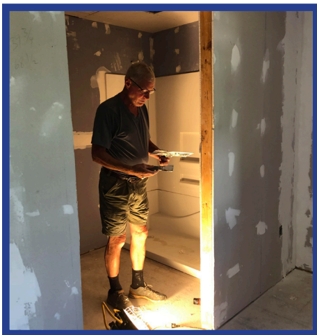
Jan Barendse from Utica, NY spackling the walls.
