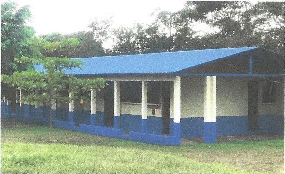
New Roof in Guatemala
