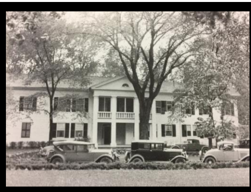
James Mason House 1931 No garage on the North side
